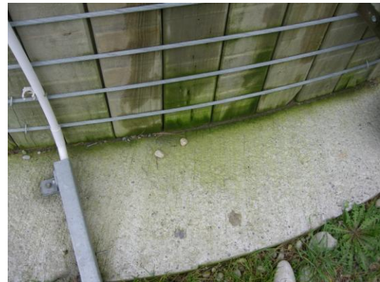
(b) Base isolation sliding of 20 mm for 180 m 3 tank near Darfield. No damage to tank.
