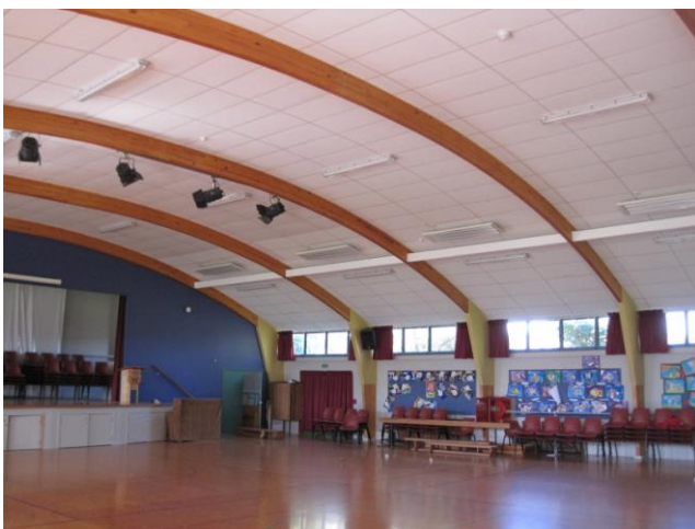
(a) No damage to curved portal frames.
