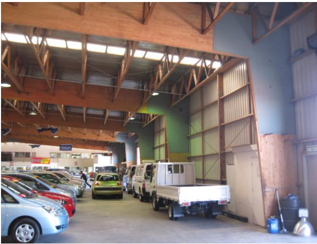
(a) Overall structure showing glulam portal frames and truss purlins.
