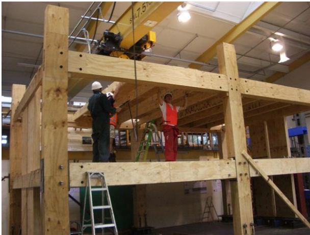
(a) Test building under construction in the University of Canterbury labs.
