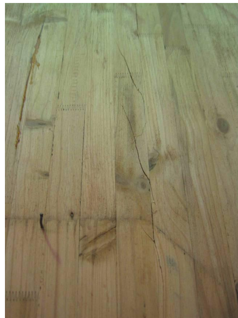
(d) Detail of shear cracks in another column of the same building.
