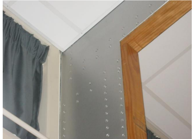
(b) No damage to nailed knee joint.
