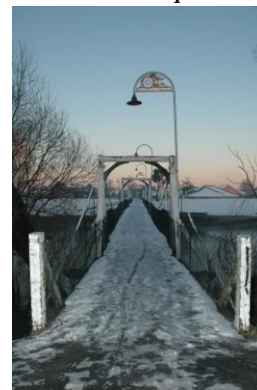
(b) Condition of repaired Mandeville Bridge as of July 2011.
