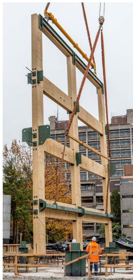
Figure 2: A post-tension timber frame being erected (courtesy of University of Canterbury)
