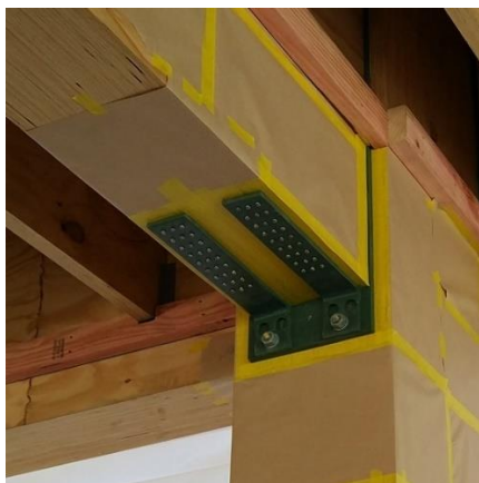
Figure 3: A beam-column connection using angle dissipaters
