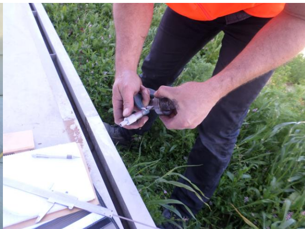
Figure 10: Measuring the diameter to check yielding of the seismic anchorage system
