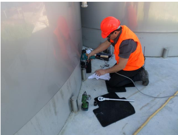
Figure 9: Removing the yielding pin mechanism of the seismic anchorage system
