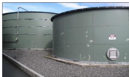
(a) No particular damage to the anchors around the tanks
