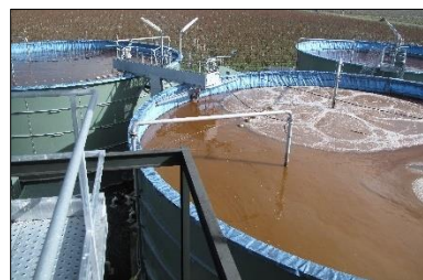
(b) Continual operation of tanks following earthquake
