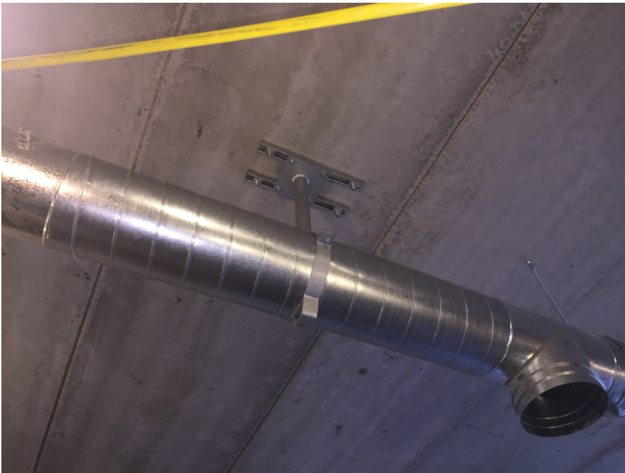
Figure 1: Cantilever post detail where Arch didn't want braces
