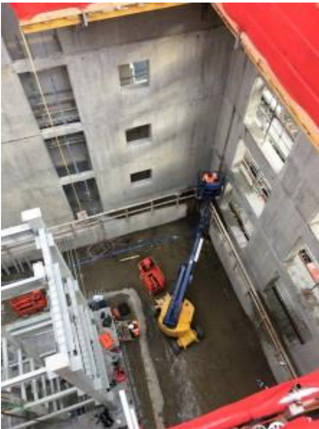
Figure 7: Jump-formwork system in action. Walls are cast a number of levels in advance of the rib-and infill floor installation. Part of the system includes a safe and secure platform for workers.
