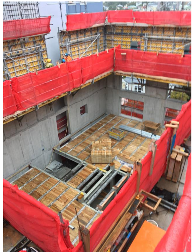
Figure 7: Jump-formwork system in action. Walls are cast a number of levels in advance of the rib-and infill floor installation. Part of the system includes a safe and secure platform for workers.
