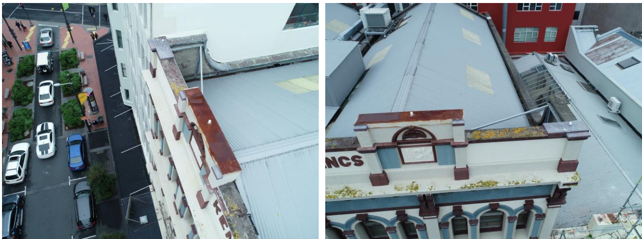
Figures 5 and 6: Images of the roof and parapet from the drone survey
