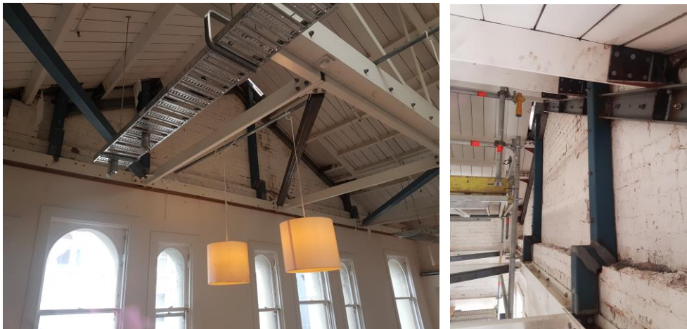
Figure 9 and 10: Steel Installation on Level 3
