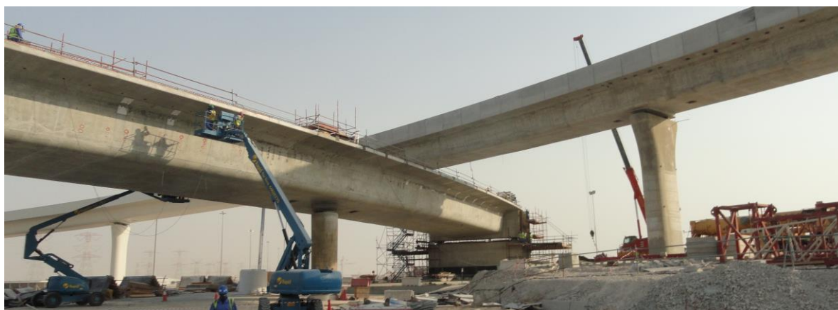
Figure 2: Construction of the new Orbital Highway in Qatar
