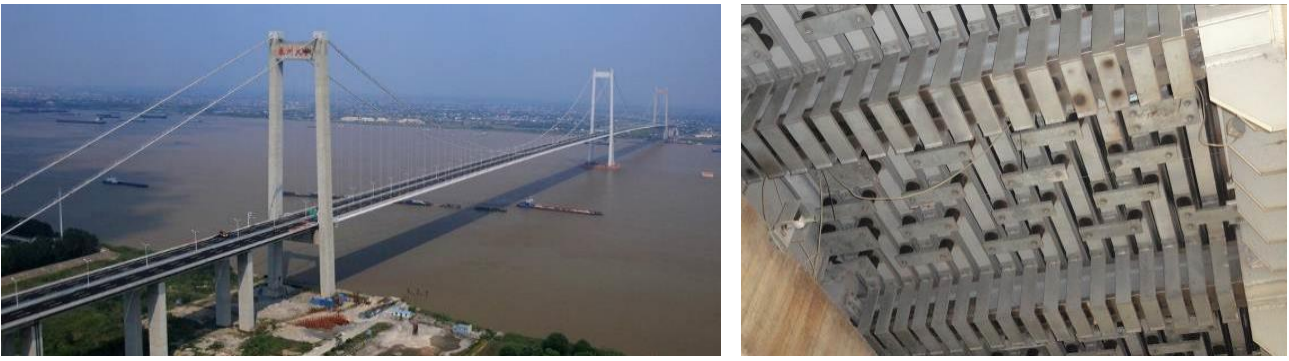
Figure 4. The Taizhou Yangtze River Bridge (left), and one of its enormous 18-gap modular expansion joints, viewed from below.
