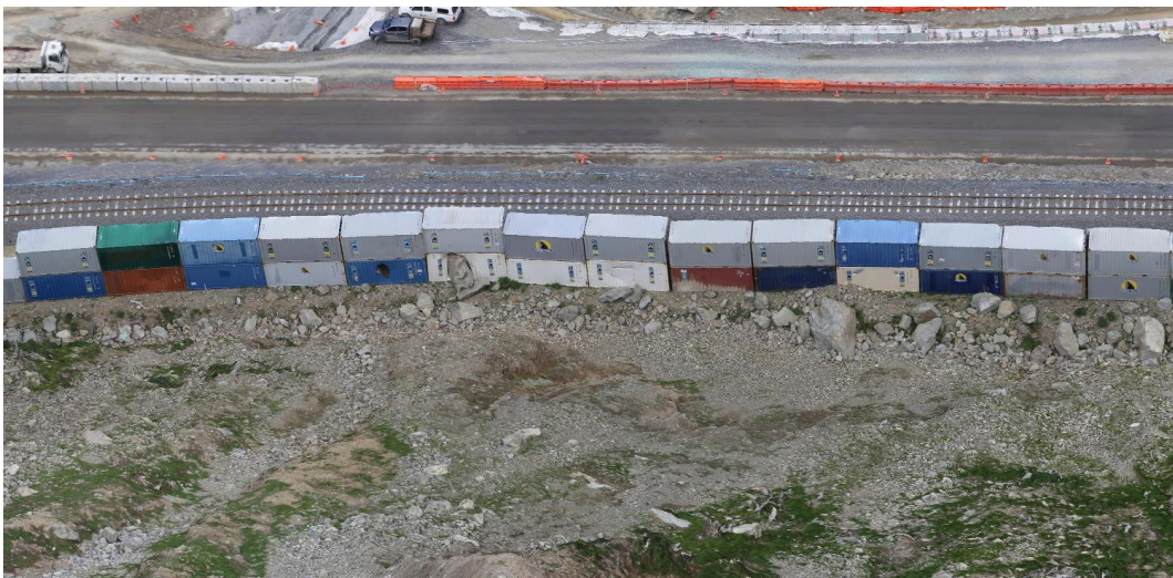
Figure 3: Boulder impacts at container wall following rock blasting
