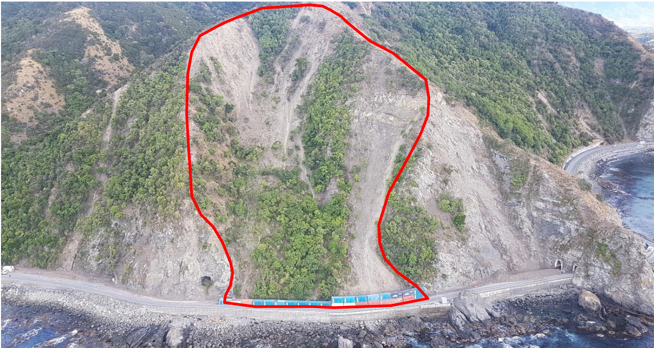
Figure 1: Earthquake damaged slopes above the coastal transport corridor, the approximate site location of SR18/19 is outlined in red
