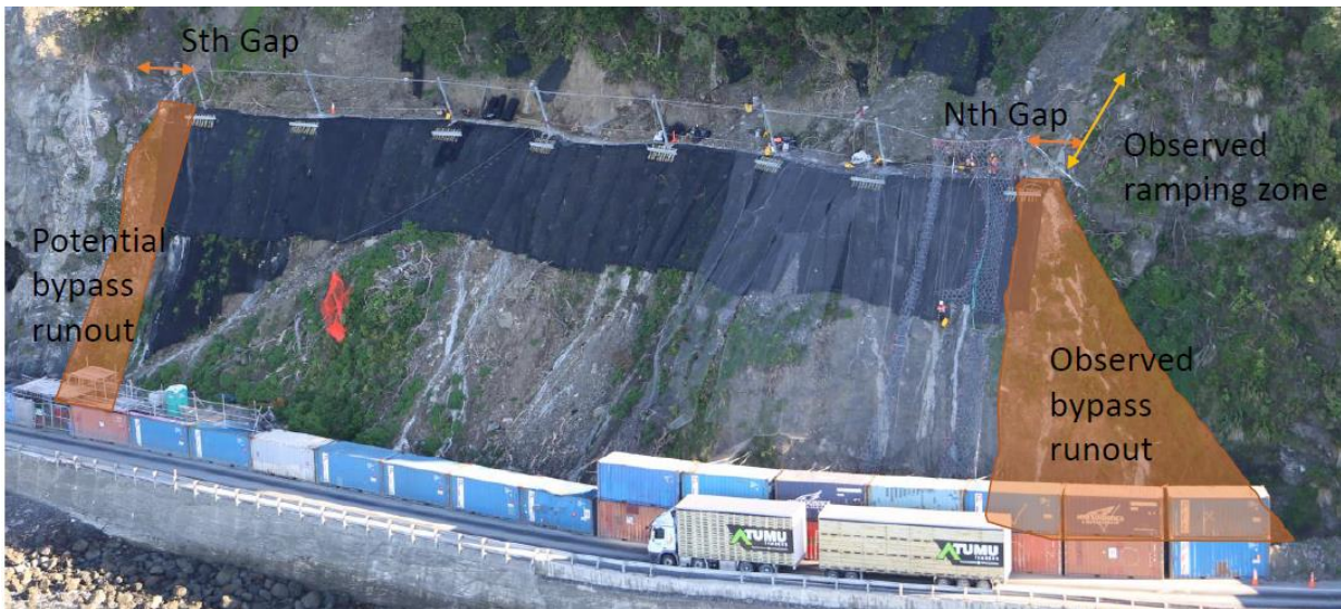
Figure 6: The mapped hazards resulting from the gaps at the edges of the hybrid fence at SR18/19
