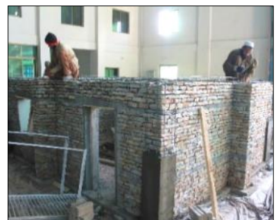
(c) RC band and splints under construction (DT 1)
