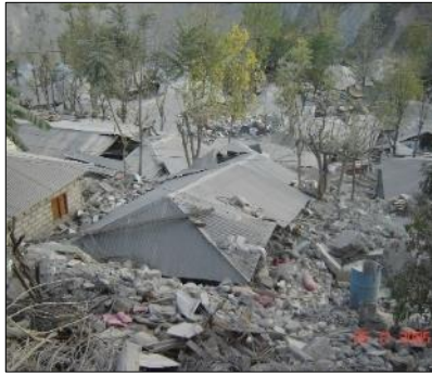
(d) Destruction of a village, during 2005 Kashmir earthquake, Pakistan
