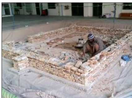
(a) Model building under construction (DT 1)
