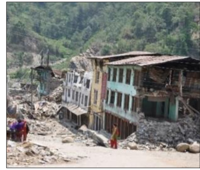
(c) Out of plane collapse of walls, destruction of top storey, 2015 Gorkha earthquake, Nepal
