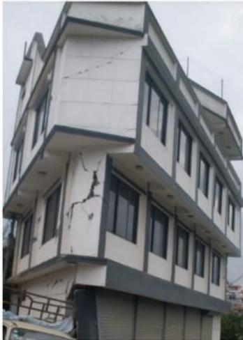
(a) Damage due to torsional effect
