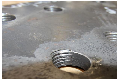
Figure 7: Threads in holes due to bearing of bolts
