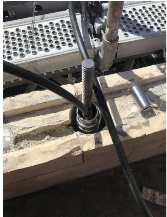
Figures 7 and 8: Rig set up for vertical drilling (left) and spiral reinforcing steel (right)
