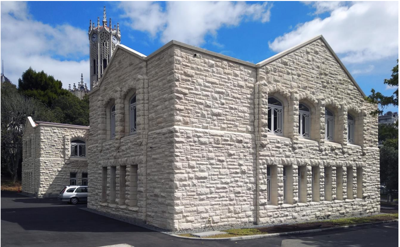
Figure 2: View of the East Wing building from South
