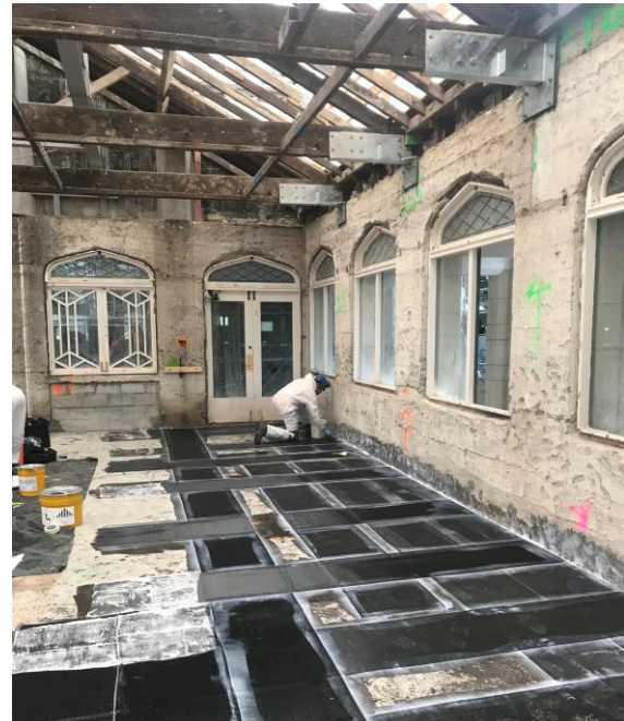
Figures 9 and 10: Substrate repair (left) and FRP on-site installation (right)
