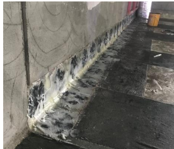
Figures 11 and 12: Perimeter skirting detail (left) FRP on-site installation to a fillet radius (right)
