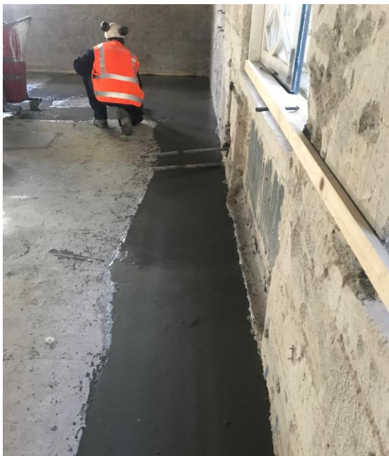
Figures 9 and 10: Substrate repair (left) and FRP on-site installation (right)
