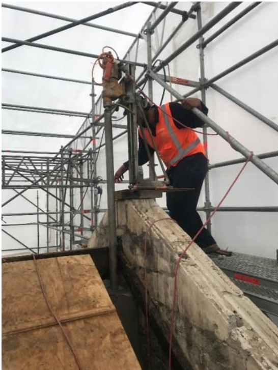
Figures 7 and 8: Rig set up for vertical drilling (left) and spiral reinforcing steel (right)
