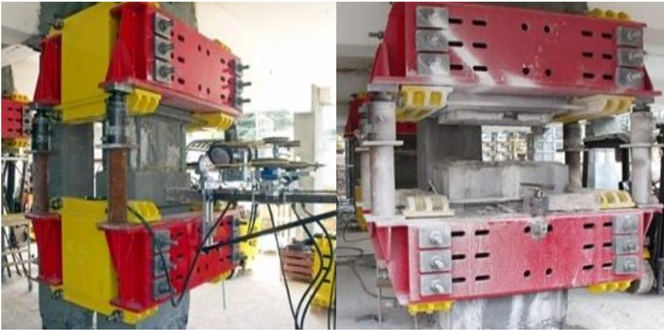
*Figure 11: Cutting machine with diamond wire (left) and removal of portion of the column (right)*
