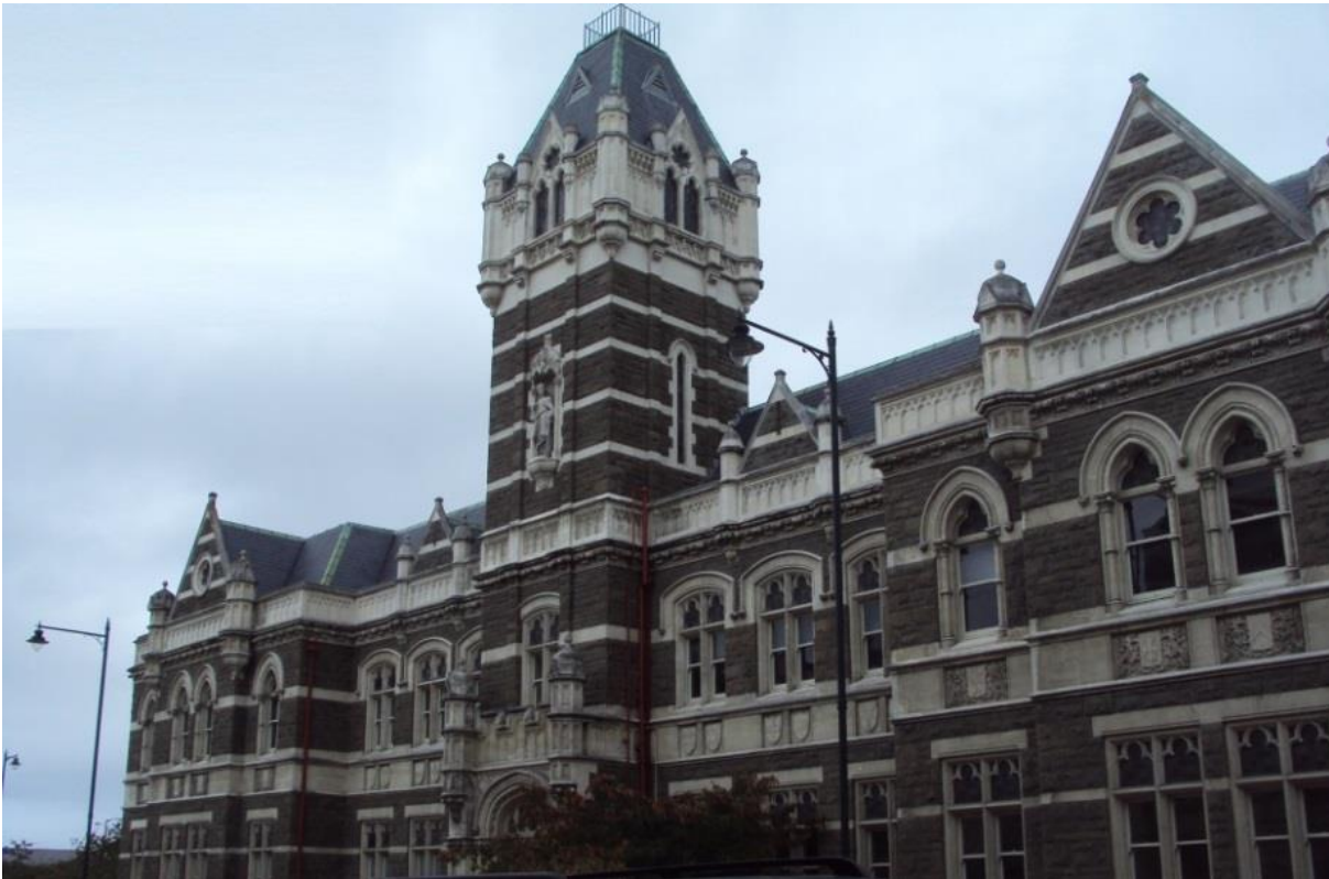
Figure 1: Photo of northern exterior of the Dunedin Law Court Building.
