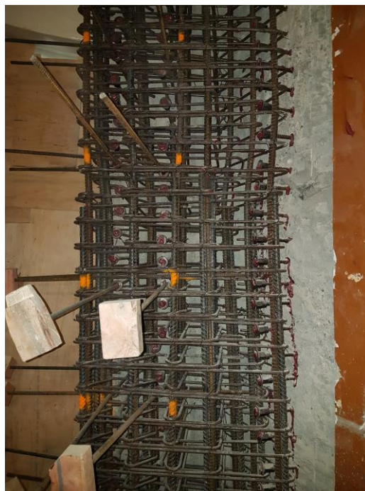
Figures 10 and 11: Looking down on the curved beam; Column reinforcing
