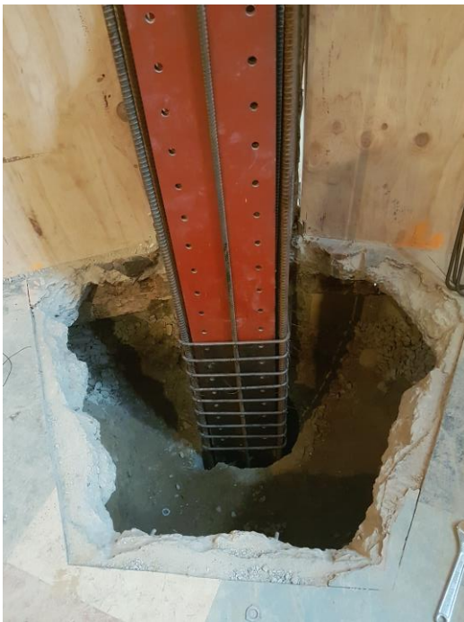
Figures 8 and 9: Steel UC and reinforcing cored into caisson; Ground water in caisson
