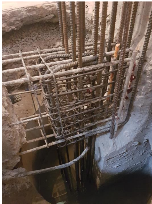
Figures 8 and 9: Steel UC and reinforcing cored into caisson; Ground water in caisson
