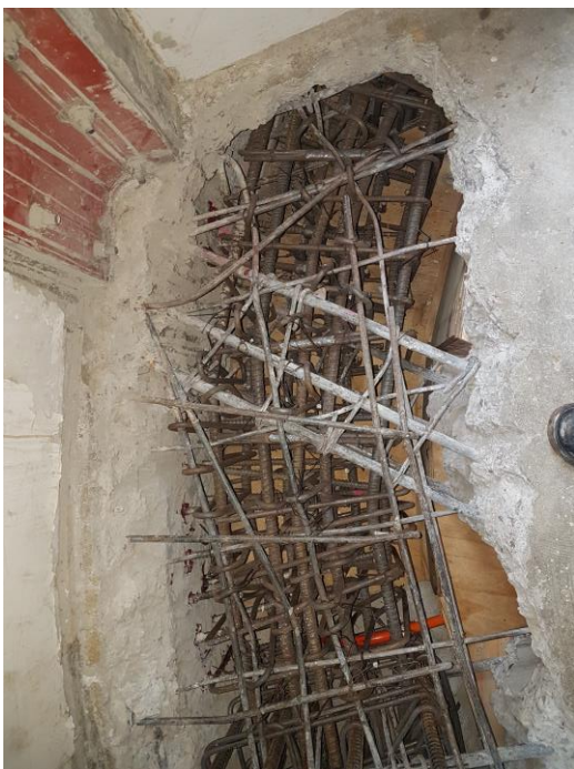
Figures 10 and 11: Looking down on the curved beam; Column reinforcing
