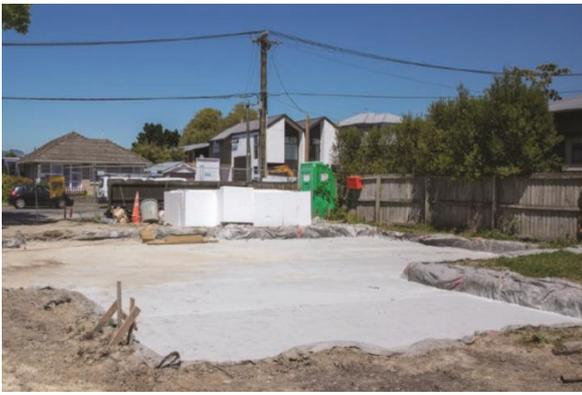
Figure 7: Completed Terefil raft
