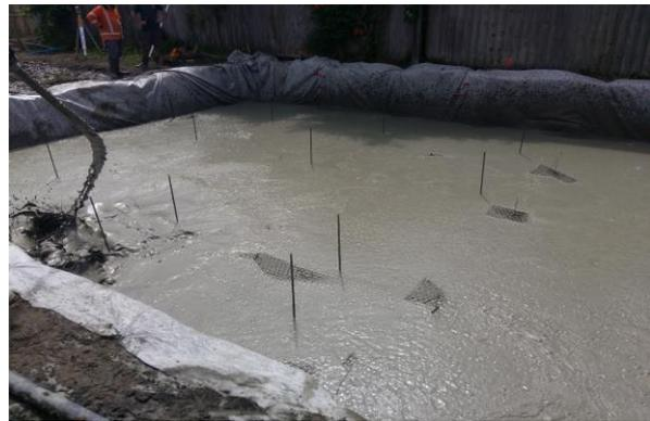
Figure 6: Terefil raft installation
