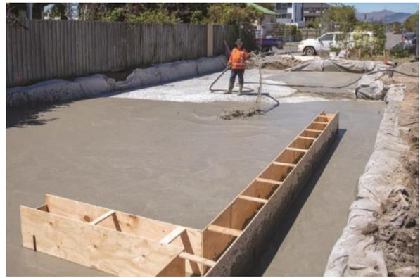
Figure 8: Formwork placed over the Terefil raft
