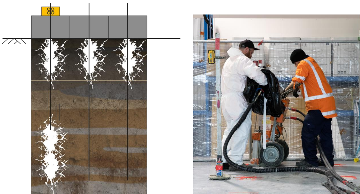
Figure 4: Capping and target improvement zones (left); and Resin Injection process (right)
