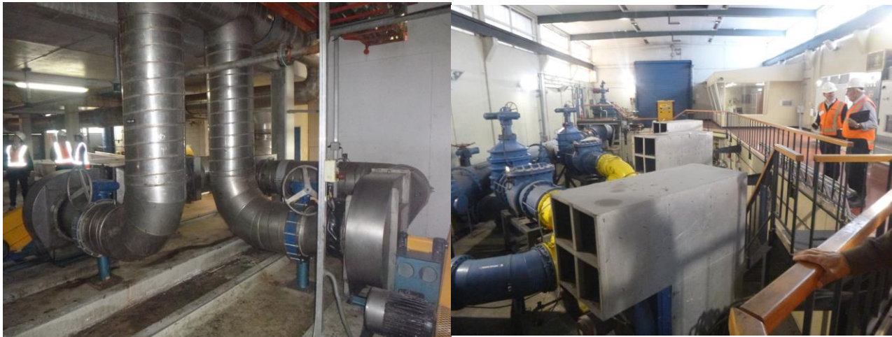
Figure 1: Photos of the Pump Station & Milliscreen Buildings (Milliscreen – Left, Pump Station – Right)
