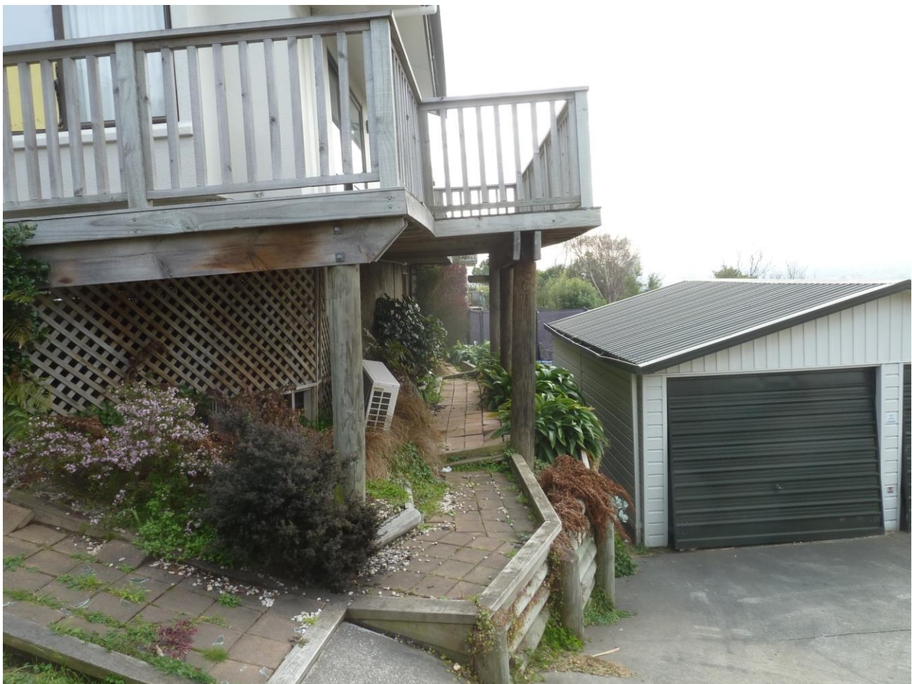
Figure 1: Tilting pole structure
