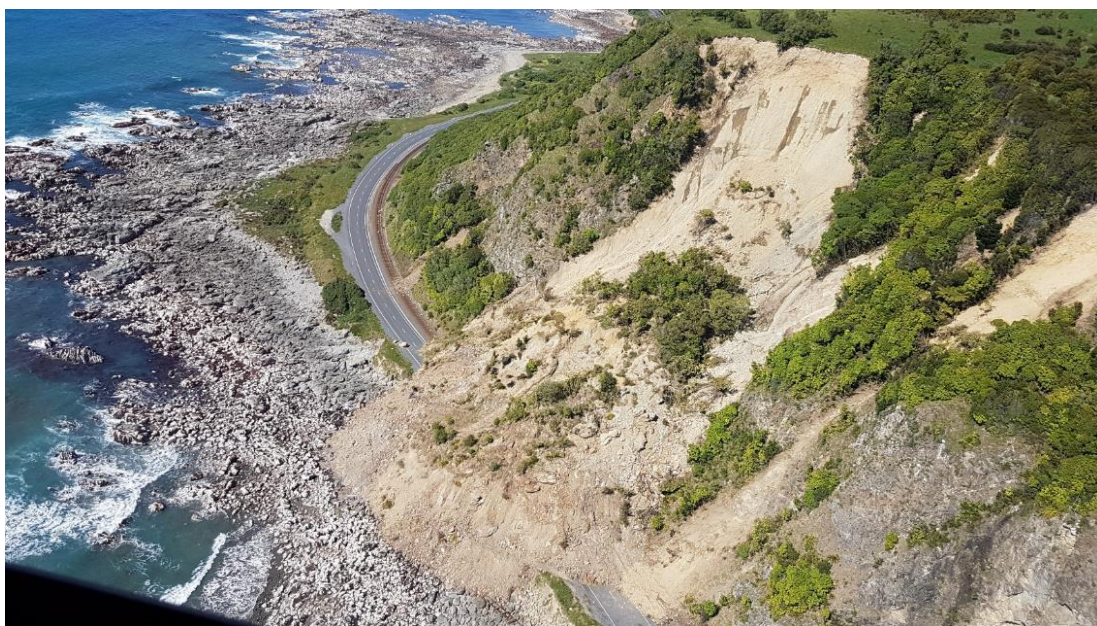
Figure 3. State highway and rail closed by large landslides in the 2016 Kaikōura earthquake, New Zealand.
