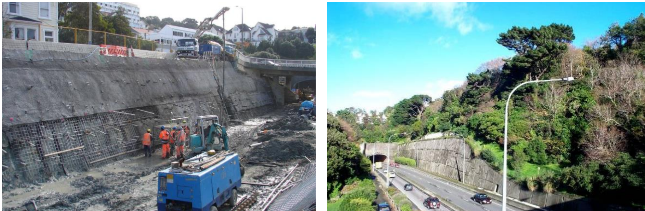
Figure 1. Soil nailed walls at Wellington inner-city bypass (left), Terrace tunnel approach walls (right)
