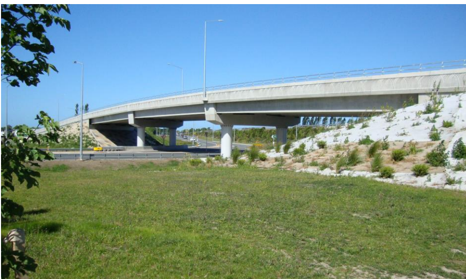
Figure 2: Wigram-Magdala Link bridge in Christchurch, New Zealand (courtesy of Jeremy Kelleher)
