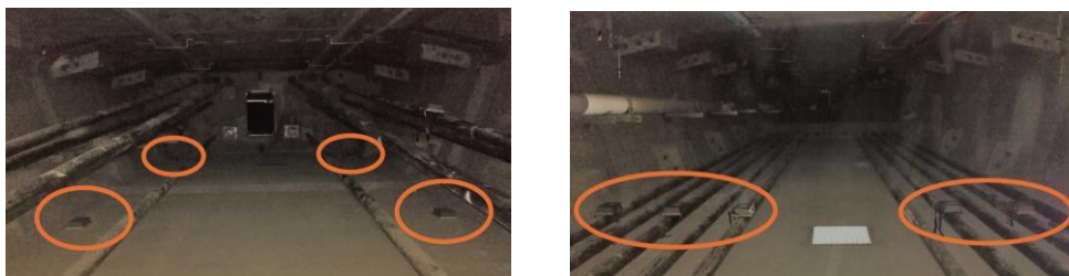
Figure 4: Bridge instrumentation using the wireless sensory system.
