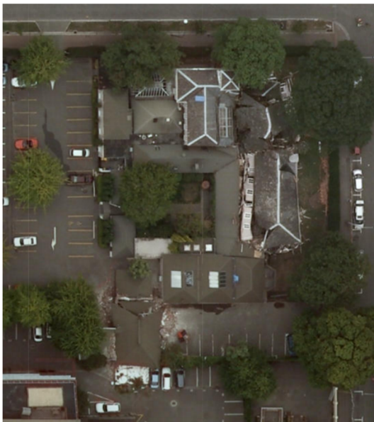
Figure 5: Aerial image of club showing collapsed Latimer wing (Canterbury maps 24 February 2011)
