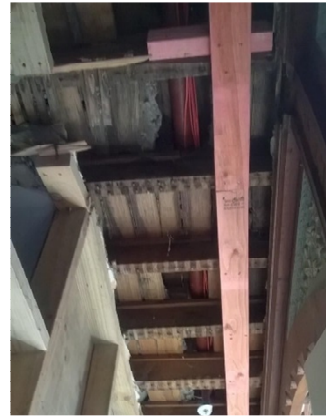
Figure 12: Underside of floor with ceiling removed. Timber battens supporting insulation visible
