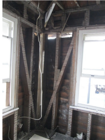
Figure 14: wall framing on first floor
