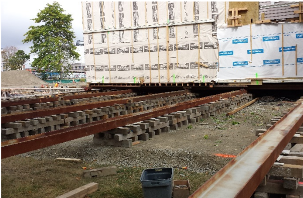
Figure 17: Shifting beams set up on dunnage
