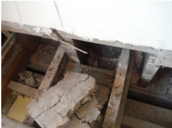
Figure 11: 1860's In floor insulation
