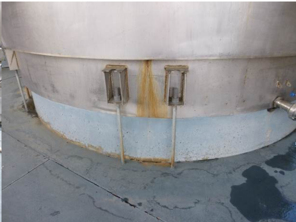
(b) Chair mounted un-necked tension anchors
