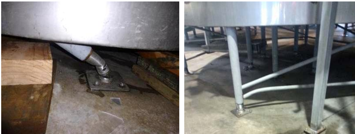
(a) Bending of un-braced leg
