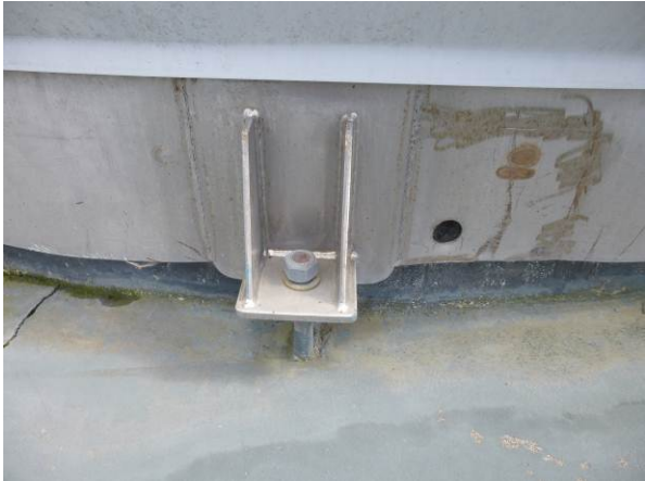
(d) Chair mounted un-necked tension anchor
