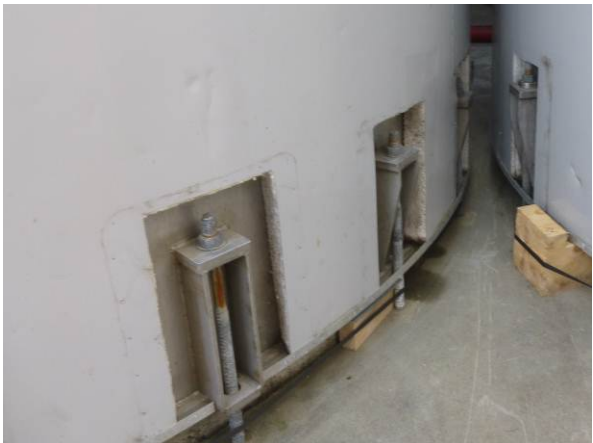
(e) Chair mounted necked tension anchors
