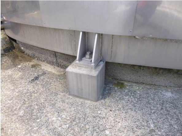
(c) Chair mounted un-necked tension anchor
