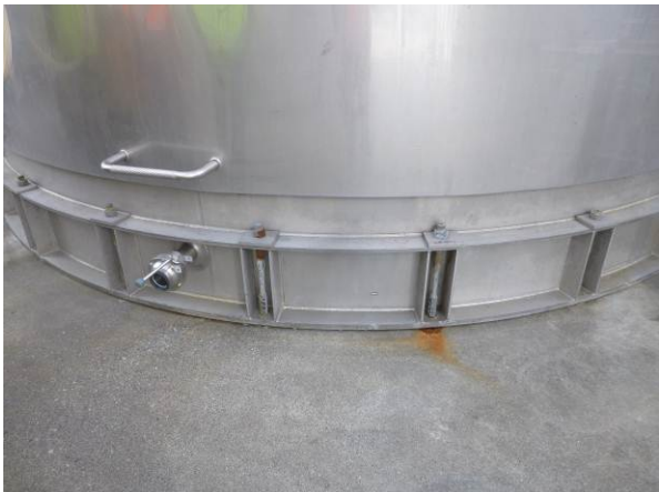
(f) Chair mounted necked tension anchors
