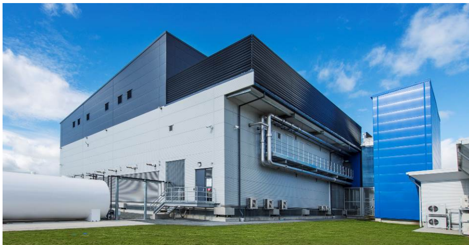
Figure 5. Completed Data Centre Facility.
