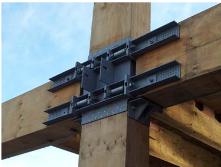
(a) Beam-column connection using rivets.
