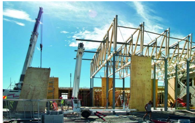
Carterton Events Center, Carterton, increased stiffness through increased section modulus.
