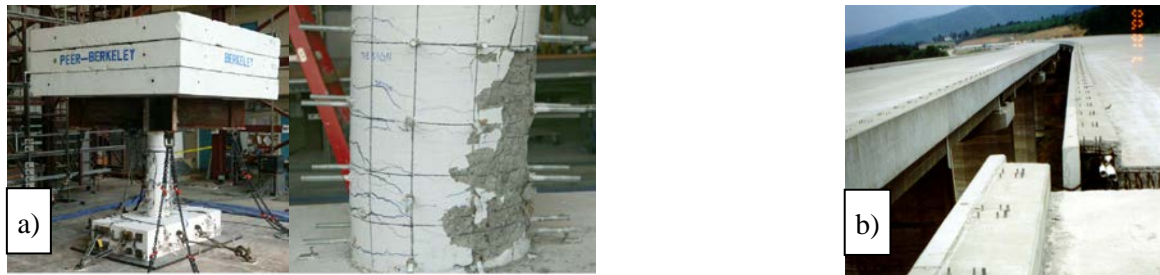
Figure 4. a) Plastic hinge formation occurring at the base of a pier designed to rock on a shallow foundation (Espinoza and Mahin 2012). b) Residual deck displacement of the seismically isolated Bolu Viaduct in Turkey following the 1999 Duzce Earthquake (Roussis, Constantinou, Erdik, Durukal and Dicleli 2002).
