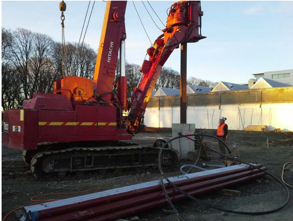
Figure 3. Excavation of typical pile.
