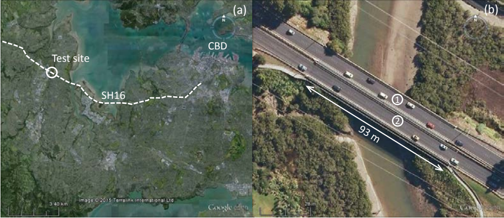
Figure 1. Test location a) in Auckland, b) close up of Henderson Creek Bridges No. 1 and 2.
