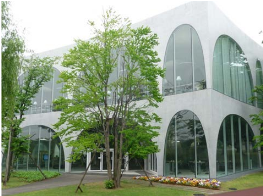
Figure 2. Tama Art University Library, Hachioji, Tokyo. Toyo Ito, 2007. Part of the two main facades. The columns touch the floors very lightly.
