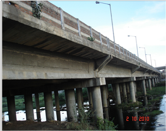
Figure 1. Longitudinal view of the study bridge
