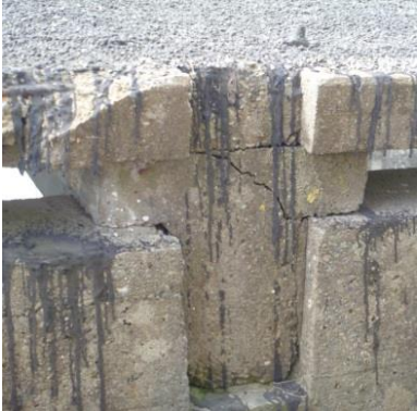
Figure 8: Joint between precast elements at Godley Head
