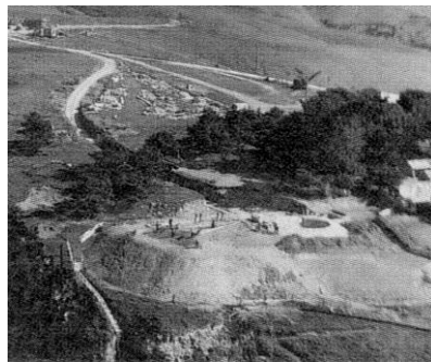
Figure 5. Construction of the bunkers at Godley Head
