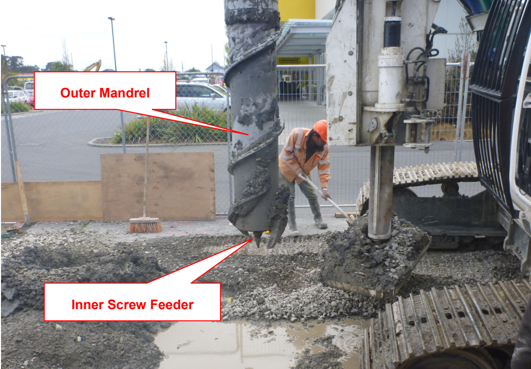
Figure 1. Stone Column Installation Rig and Screw Tool
