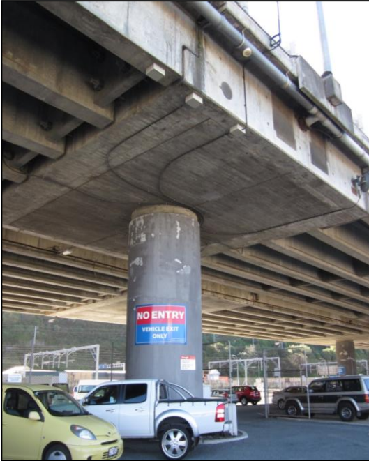
Figure 4. Accelerometers and GPS instruments on Pier 14 cap.
