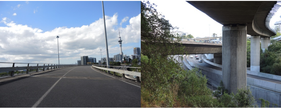
Figure 1. Views of the Nelson St off-ramp bridge
