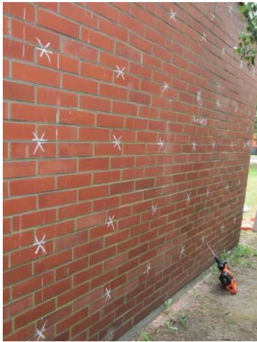
Figure 5. Marked brick veneer showing tie layout
