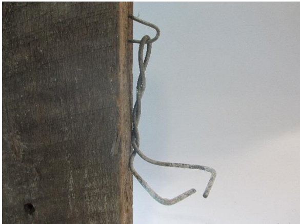
Figure 11. Detail of wire tie attached to face of stud
