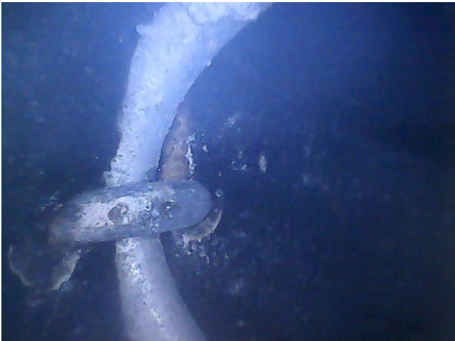
Figure 8. Wire tie attached to the face of a stud
