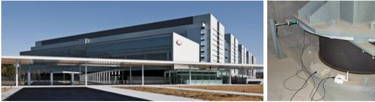
Figure 1. Example of base isolated buildings in Japan: Takeda Pharmaceutical Company Shonan Research Center, Fujisawa City, Kanagawa
