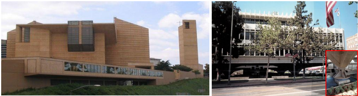
Figure 2. Example of base isolated buildings in the US: Cathedral of Our Lady of Los Angeles, Los Angeles, CA (left), Municipal Service building, Glendale, CA (right)
