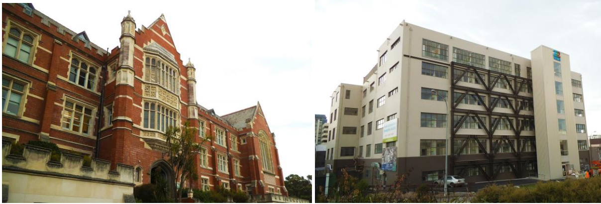
Figure 2. Shear walls hidden inside the building, keep the existing façade untouched (left). Braced frames exposed on the façade of the building (right).
