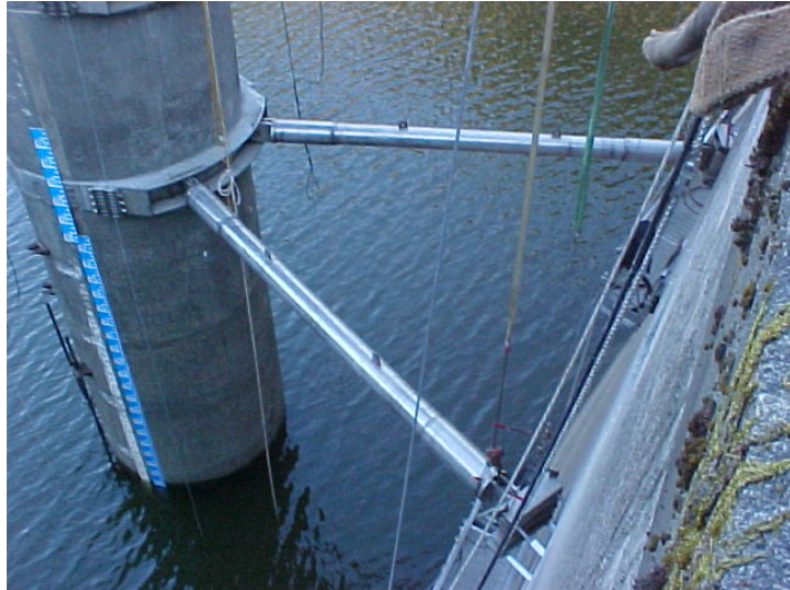
Figure 6. Casad Dam, Bremerton, WA, US
