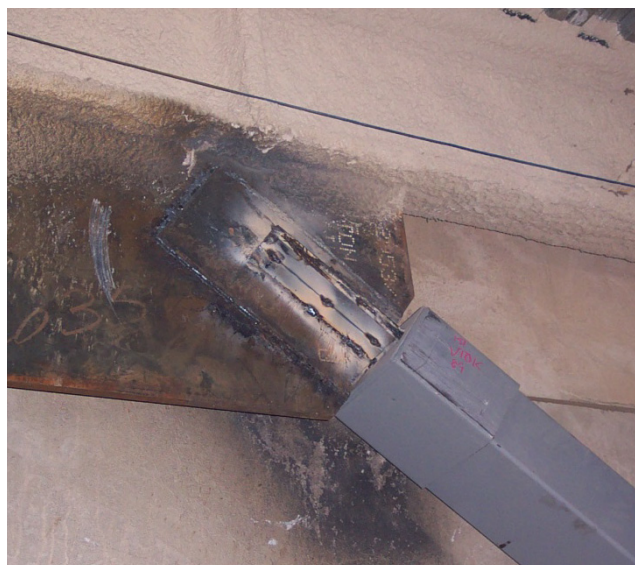
Figure 7. Data Centre Retrofit Utilizing Existing Gusset Plates
