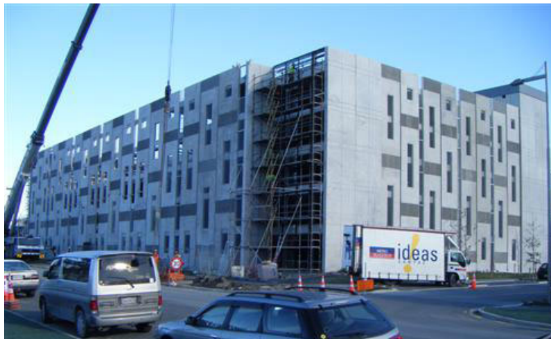
Figure 3. Hazeldean Car Park, Christchurch, NZ
