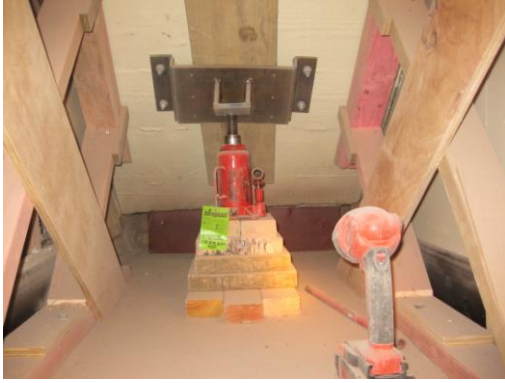
Figure 11: Cab access stair jacking
