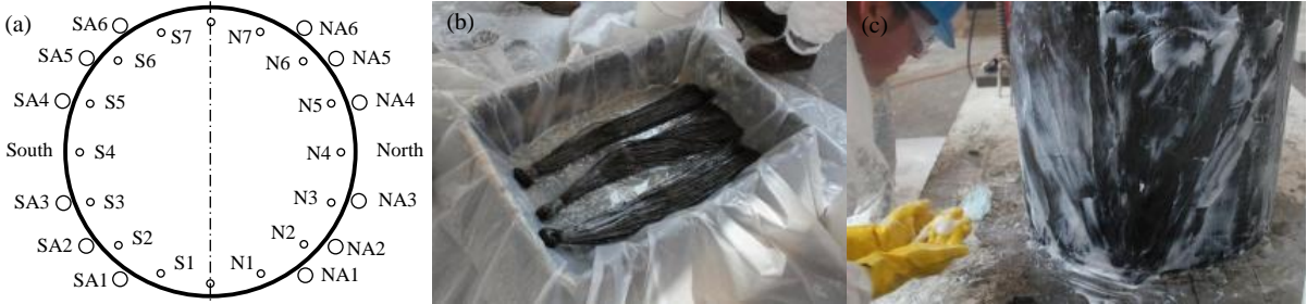
Figure 1: Configuration (a), saturation (b) and installation (c) of carbon fiber anchors
