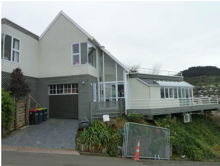
Figure 7. House on Sloping site with horizontal and vertical irregularities and differing foundation types.
