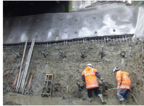
Figure 5. Mohaka Bridge south abutment strengthened using post-grouted soil nails
