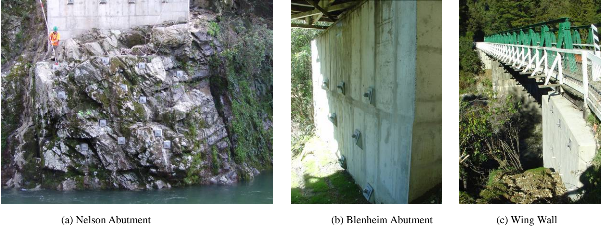
Figure 3. Rock anchor strengthening of abutments at Pelorus Bridge
