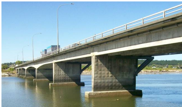
Figure 8. Cobham Bridge across the Wanganui River
