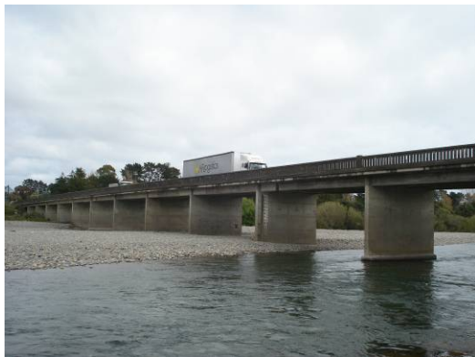
Figure 6. SH1 Otaki River Bridge and its north abutment
