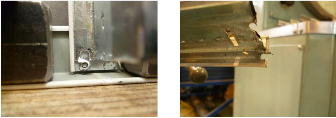
Figure 7. Failure mode in the rivet connection between the main beam and the wall angle
