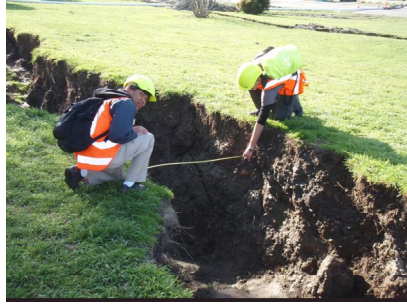
(a) Measuring crack width
