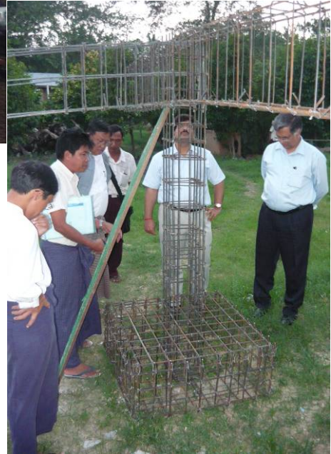
(c) A mock-up joint at MES
