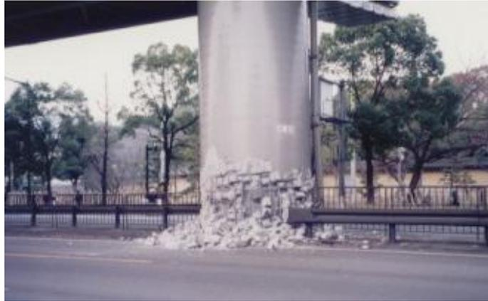
Figure 1: A damaged column after the 1995 Kobe earthquake. (Courtesy of UC Davis archives.)
