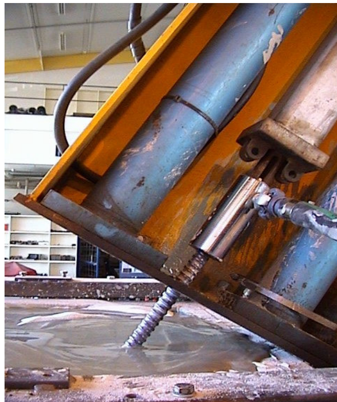
Figure 7. Installation of inclined micropiles.
