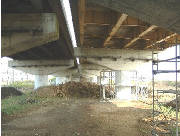
Figure 3. Twin bridges on National Highway No. 8 over the railway in Ojiya
