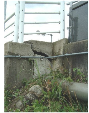
(c) Horinouchi Bridge
